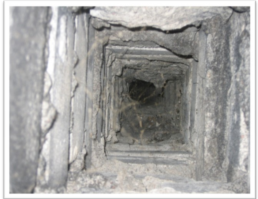
Airing through the windows in case of the clogged ventilation
