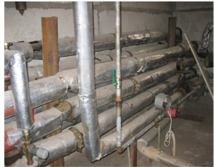
Old Heating System (example of an old heat exchanger for hot water)
